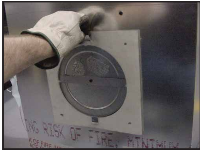
Figure 9.6 Fold the tabs toward the center of the seal cap (90°) and remove the insulation gasket.
